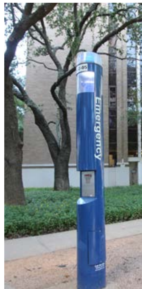
Emergency telephone pedestal phones provide direct access to UT Police.
